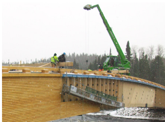
FIGURE 13 – Pont Maicasagi, QC (Source : Nordic Structures)
