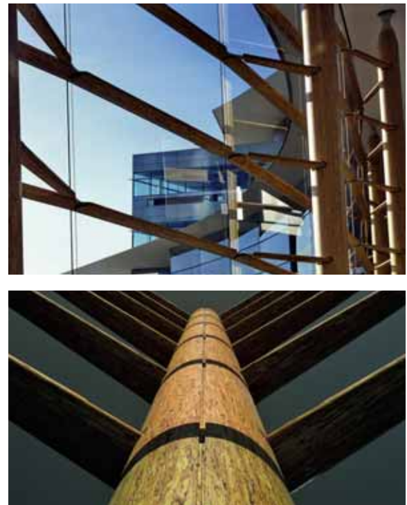
FIGURE 13 • Bois PSL au centre commercial Central City à Surrey (C.-B.) (photos : StructureCraft Builders)
