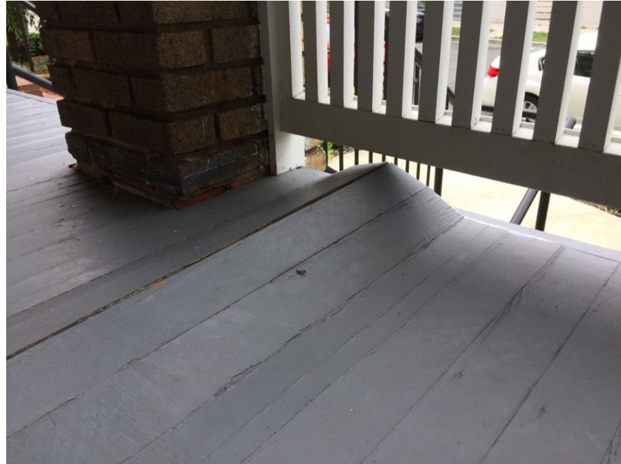
Dealing with a wooden porch that buckles when it rains - The Washington Post
