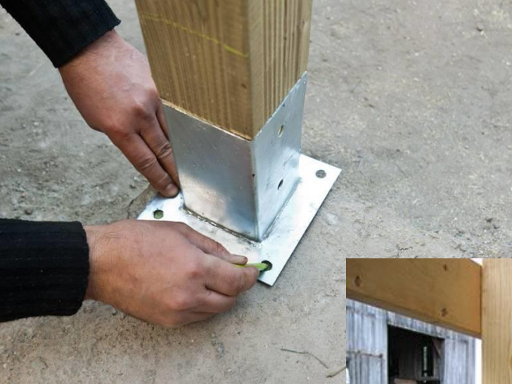
How to anchor post to concrete | HowToSpecialist - How to Build, Step by Step DIY Plans
