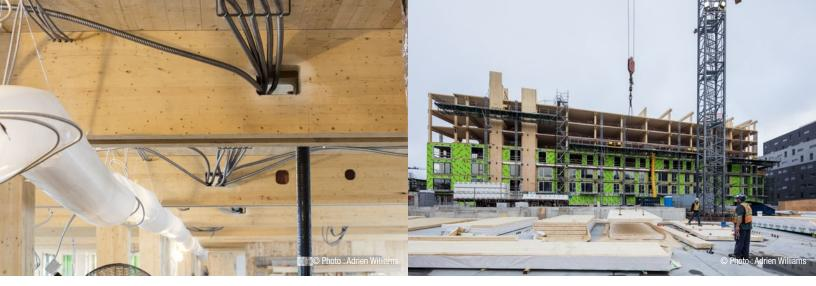
Beams with pre-drilled holes for machinery
