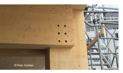
Self-tapping screws are used to secure the beams in case of fire
