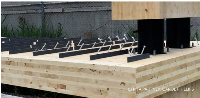
MOCK-UP OF THE SLAB USED IN THE CONSTRUCTION OF THE BUILDING
