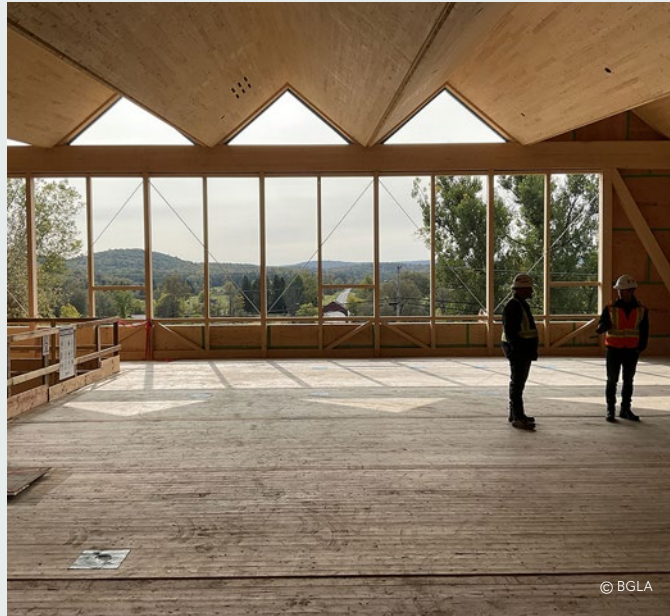
INSIDE THE LA PÊCHE TOWN HALL BUILDING SITE
