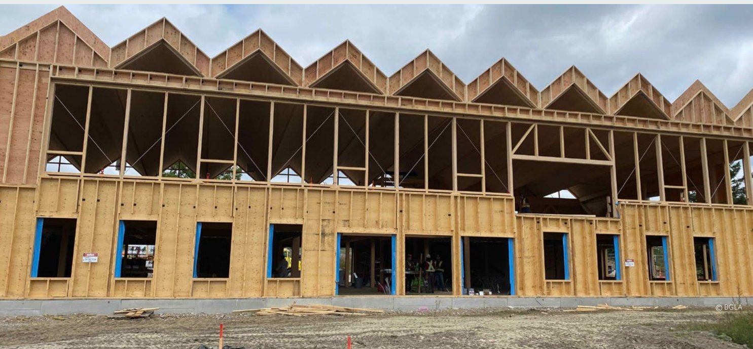
OUTSIDE THE LA PÊCHE TOWN HALL BUILDING SITE
