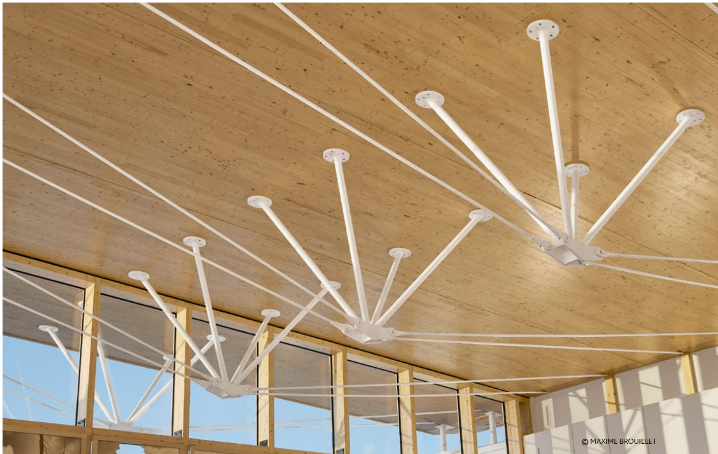
INTERIOR VIEW OF THE CHIBOUGAMAU-CHAPAIS AIR TERMINAL
