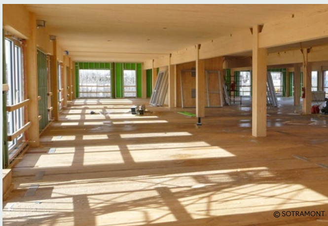
INSIDE THE TOD ECO-HOUSING BUILDING SITE
